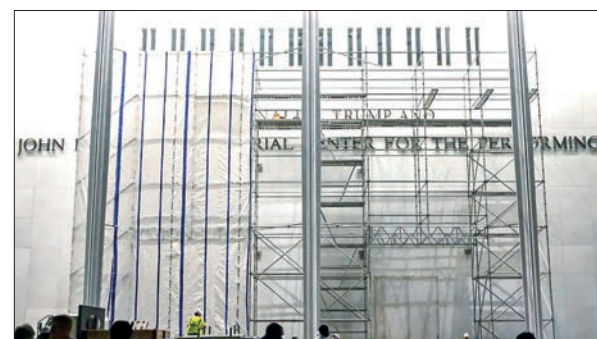
Workers build scaffolding and hang flame retardant tarps near the signage for the “Donald J Trump and John F Kennedy Memorial Centre for the Performing Arts” in Washington, DC, early on 13 June 2026. PHOTO: ALEX WROBLEWSKI/AFP
